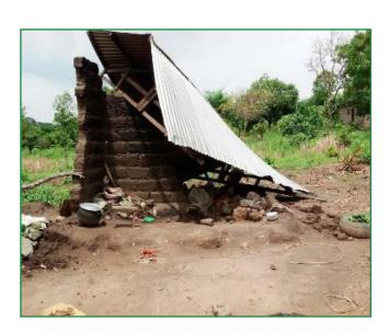
Houses destroyed due to vibrations from quarry blasting
